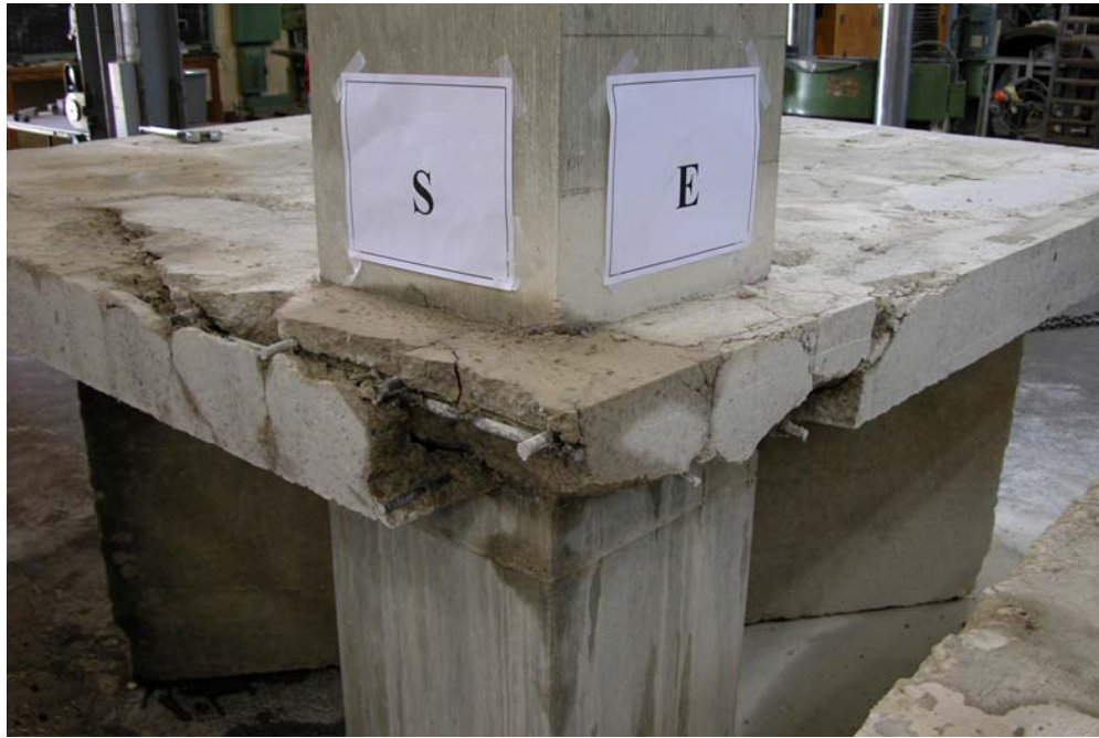
Figure B.2: Failure surface of Specimen LG0.5.
