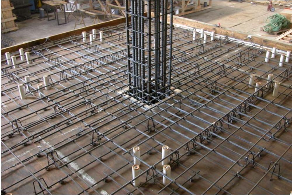
Figure 2.28: Steel cages and slab forms (Specimen LG1.0).
