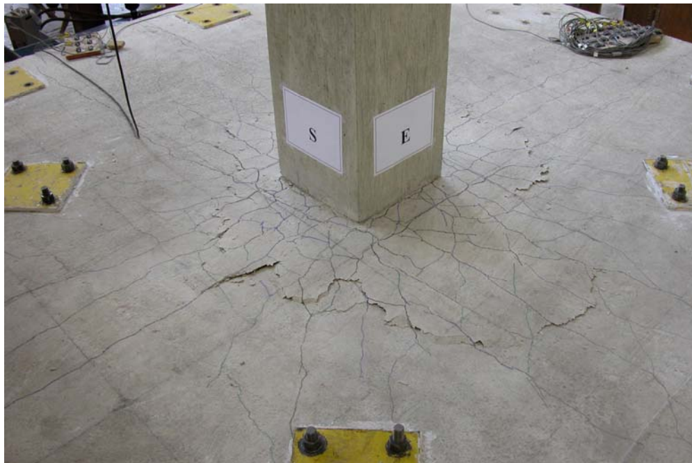
Figure B.3: Failure pattern of Specimen LG1.0.
